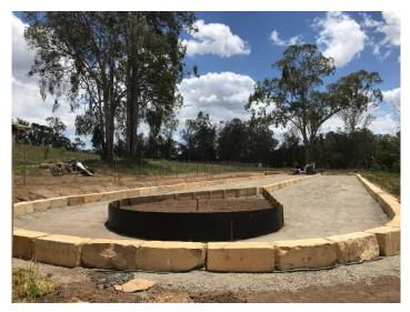
The structural part of the new 65m x 12m raceway pond was completed by 11 December. The image at left shows the outside wall and the centre wall built using 1m (L) x 400mm (W) x 400mm (H) sandstone blocks, each weighing 600kg.
